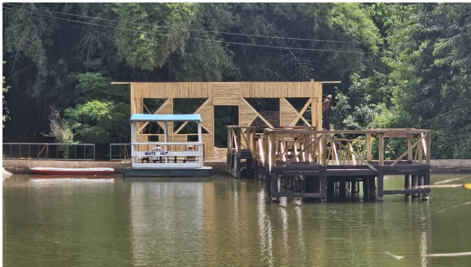
Photo 21 Visitor banda under construction at Pugu-Kazimzumbwi
